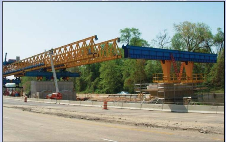
The first guideway span erection, taking place on the Dulles Connector Road at the Chain Bridge Road overpass. Photo by Stephen Barna, Dulles Corridor Metrorail Project
