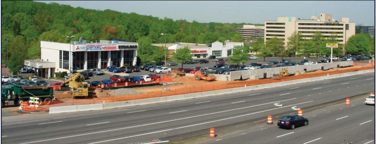
Retaining walls on Route 7, necessary to build up the service roads to the same grade as Route 7 for lane shifting. Photo by Stephen Barna, Dulles Corridor Metrorail Project
