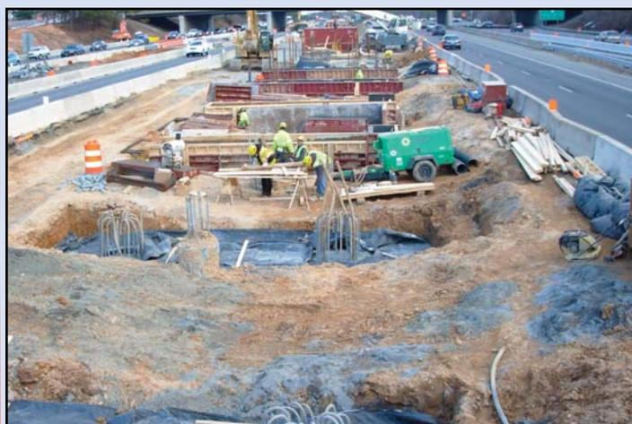
Caissons under construction for the foundations of the Wiehle Avenue Metro Station site. Photo by Dulles Corridor Metrorail Project
