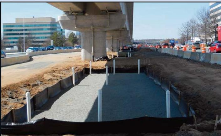
UNDER THE TRACKS: This large hole is a basin construction happening beneath the aerial guideway in the Route 7 median looking west from Gosnell Road where drain piping and a gravel bed are being installed prior to placement of soils. Photo by Stephen Barna, Dulles Corridor Metrorail Project
