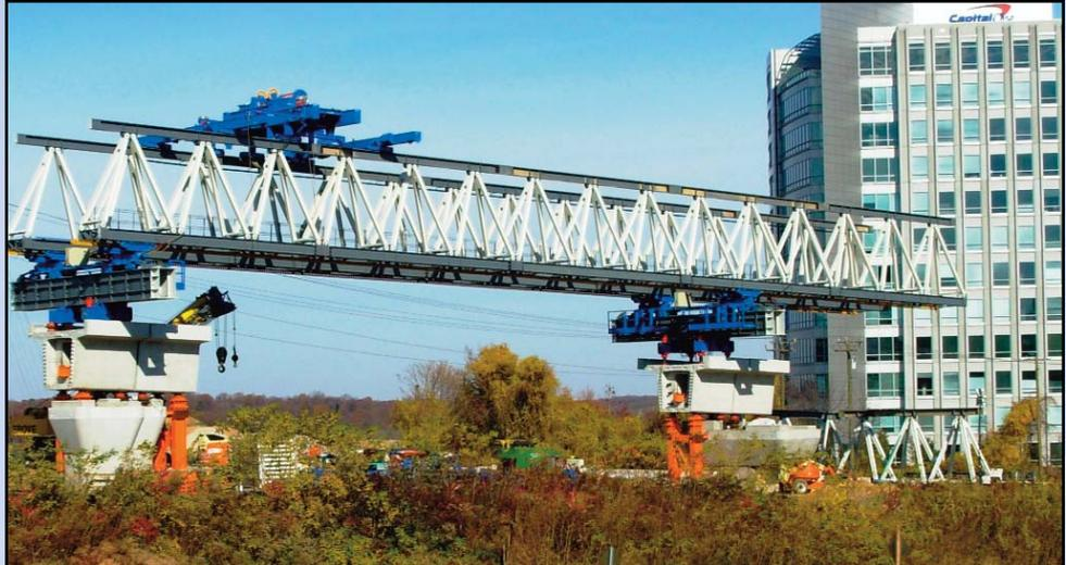
OVER THE BELTWAY: Construction begins to bring the Dulles Metro tracks over the Beltway in Tysons Corner using a white truss. Photo by Chuck Samuelson, Dulles Corridor Metrorail Project
