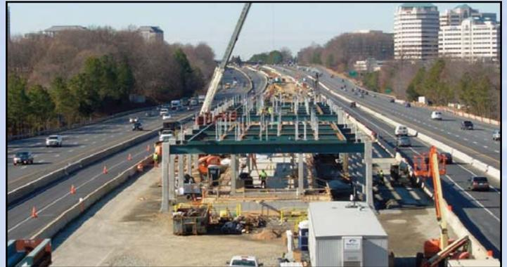
STATION CONSTRUCTION: Crews continue to work on the structural steel for the mezzanine. Photo by Chuck Samuelson, Dulles Corridor Metrorail Project
