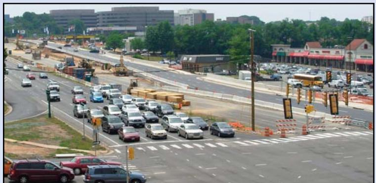
Pedestrians have a little bit of help crossing the widened Route 7 at Westpark Drive/Gosnell Road because crews have installed new traffic signals to allow walkers to walk halfway across, stop and press a signal button to get a green light to continue to cross the road. Site preparations for construction of the Tysons Central 7 Metrorail Station are visible in the median. *Photo by Stephen Barna, Dulles Corridor Metrorail Project*
