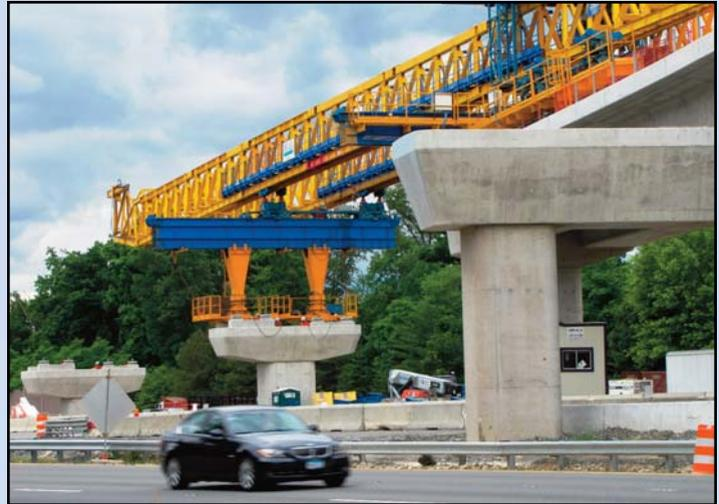
MOVING TOWARD COMPLETION: Crews continue to use a huge bright yellow horizontal crane to build the bridges for rail from Route 7 to the median of the Dulles International Airport Access Highway/Dulles Toll Road. This work is expected to be completed in July. Photo by Chuck Samuelson, Dulles Corridor Metrorail Project
