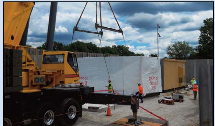
POWERING THE SILVER LINE: A large crane moves components of a traction power substation from heavy haul trucks at Magarity Road and Olney Road in the McLean/Falls Church area. Photo by Stephen Barna, Dulles Corridor Metrorail Project
