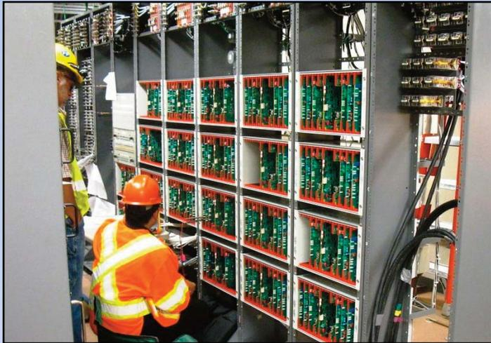
CONTROLLING THE TRAINS ON THE SILVER LINE: Crews perform static testing on automatic train control equipment in the train control room at the Wiehle-Reston East Station. Photo by Geoff Griffith, Dulles Corridor Metrorail Project continued from page 1
