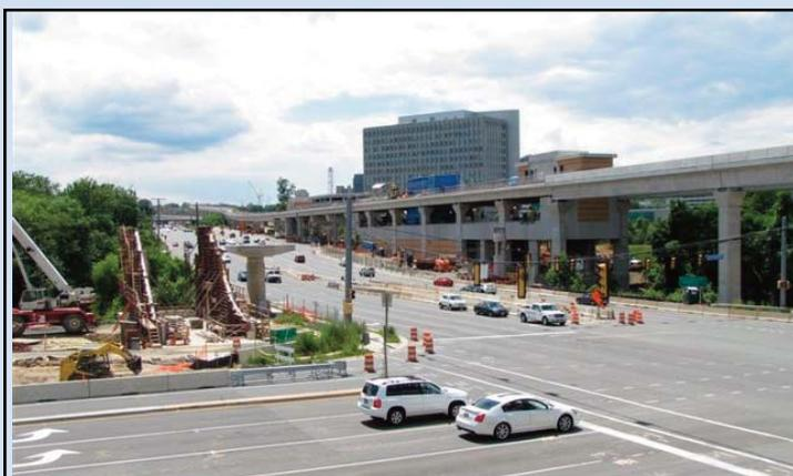
GETTING TO THE MCLEAN (formerly Tysons East) STATION: Walls are under construction for the pavilion which will provide pedestrian access from the southwest side of Route 123 to the station. Photo by Stephen Barna, Dulles Corridor Metrorail Project
