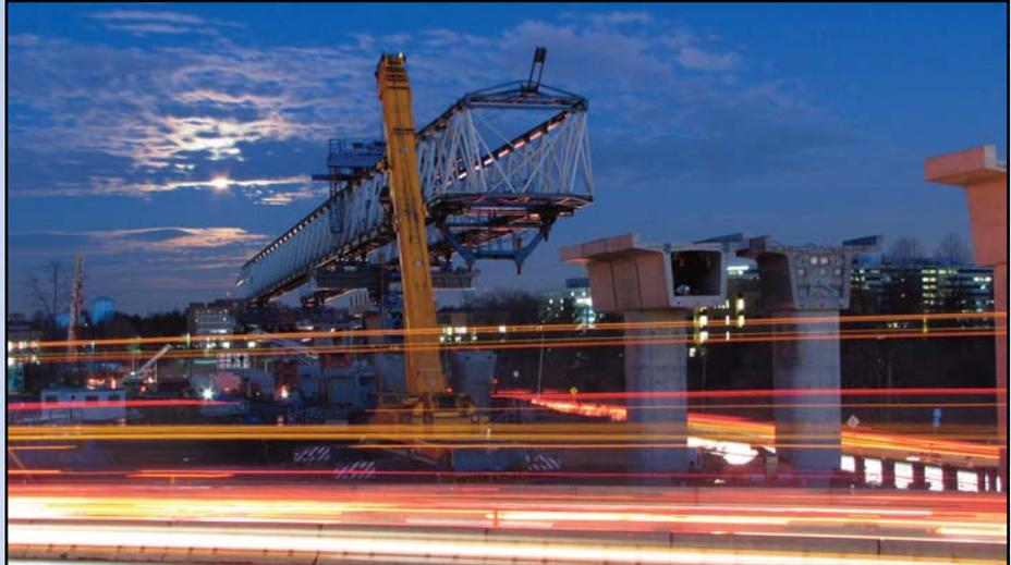
**READY TO CROSS I-495:** This horizontal crane, or truss, is being used to build segments between piers to create bridges to carry Dulles Rail trains across the Capital Beltway. *Photo by Chuck Samuelson, Dulles Corridor Metrorail Project*
