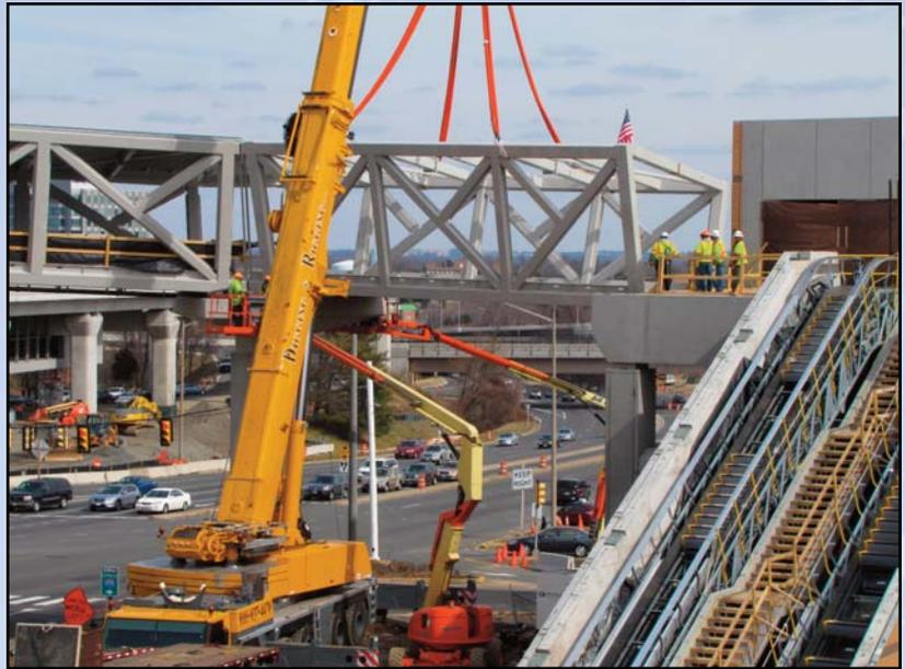
IN PLACE AT TYSONS CORNER STATION: Crews complete the installation of the last segment of the pedestrian bridge that connects the Tysons Corner Station with the pedestrian pavilion near Tysons Corner Center. Framework for pavilion escalators is at right. *Photo by Chuck Samuelson, Dulles Corridor Metrorail Project*
