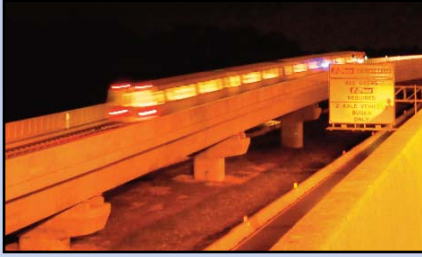
DYNAMIC TESTING: Throughout the Phase 1 alignment, testing of the Automatic Train Control continues. Photo by Stephen Barna, Dulles Corridor Metrorail Project
