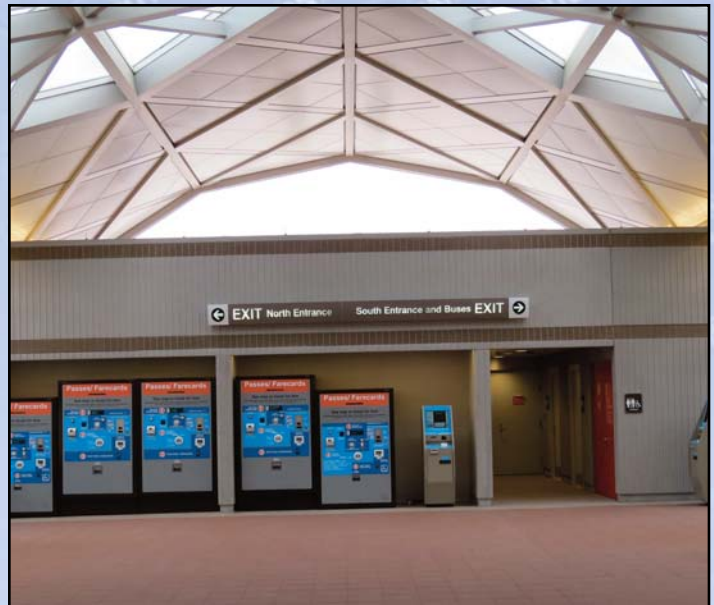
ALMOST READY FOR CUSTOMERS: Fare card machines are in place at the Wiehle-Reston East Metrorail Station. Photo by Chuck Samuelson, Dulles Corridor Metrorail Project
