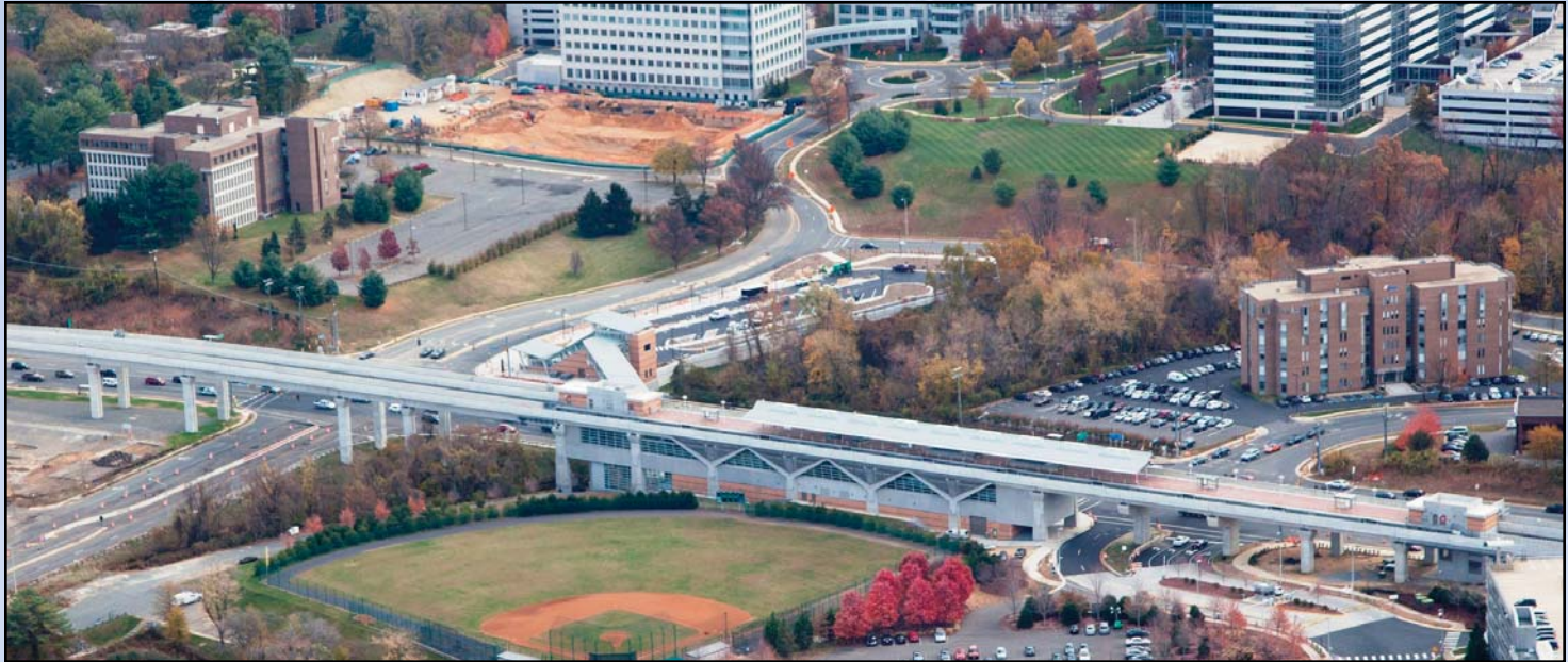
A VIEW FROM ABOVE: Virginia Department of Transportation Photographer Trevor Wrayton captured this view of the McLean Station and the aerial guideway along Route 123 near the Dulles Connector Road/Toll Road. Capital One is at the lower right. The ball fields are on the grounds of Capital One.
