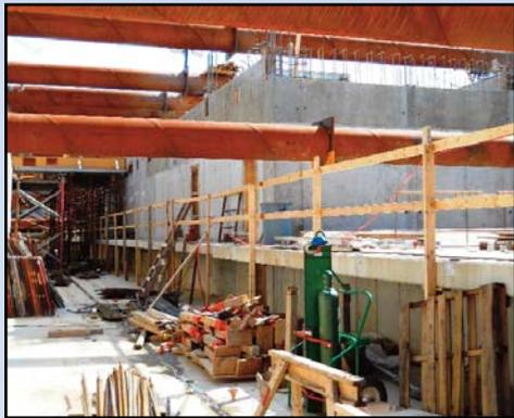
SUPPORT SYSTEMS: Platform walls and deck and the train control room and walls of an ancillary room are complete along a section of trackway. Photo also shows installation of towers for a fan room. Photo by Stephen Barna, Dulles Corridor Metrorail Project
