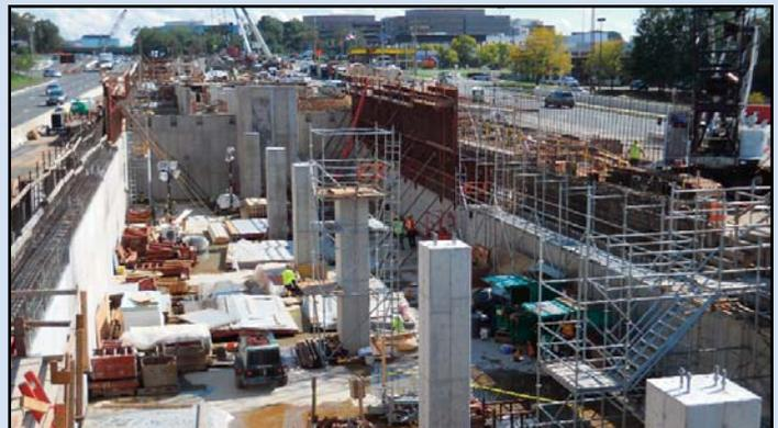
POWER FOR RAIL: Pictured is Traction Power Substation 5 at the Tysons Central 7 Metrorail Station. It is being built below the station platform deck. Retaining walls on both sides are in various stages of completion in preparation for structural steel framing. Photo by Stephen Barna, Dulles Corridor Metrorail Project
