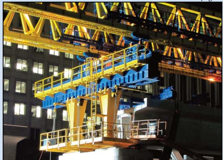
ABOVE ROUTE 7: Crews work to build bridges in the median of Route 7, using a large yellow and blue horizontal crane to lift concrete segments into place. Photo by Chuck Samuelson, Dulles Corridor Metrorail Project
