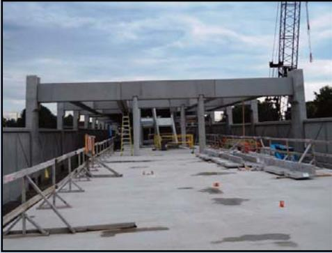
AT WIEHLE AVENUE: Looking east from the west end of the station platform, the concrete cladding of the steel framing for the mezzanine is complete. Photo by Stephen Barna, Dulles Corridor Metrorail Project
