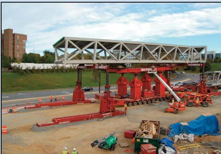
**PREPARING THE MOVE:** The transport is moved into position under the pedestrian bridge. Each tire on the transport is able to move 360 degrees, greatly increasing its maneuverability. *Photo by Leslie Periera, Dulles Transit Partners*
