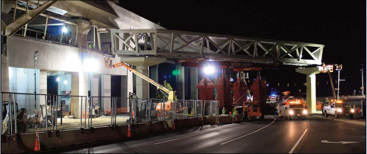
**IN PLACE:** The first section of the pedestrian bridge across Route 123 into the McLean Station, aka Tysons East Metrorail Station, is put into place. At left, workers inside the station itself watch as crews connect the bridge section to the station. *Photo by Chuck Samuelson, Dulles Corridor Metrorail Project*
