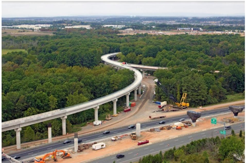
*The elevated aerial guideway at the north end of Dulles International Airport will carry trains into and out of the new rail maintenance yard and into the median of the Dulles Greenway, where the trains will return to at-grade ballasted track. Photo by: Jennifer Alcott, Capital Rail Constructors*
