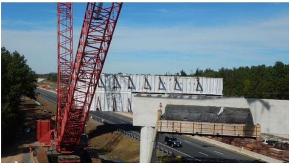
*A large concrete span (straddle bent) is constructed over the eastbound lanes of the Dulles Greenway. Photo by: Jennifer Alcott, Capital Rail Constructors*
