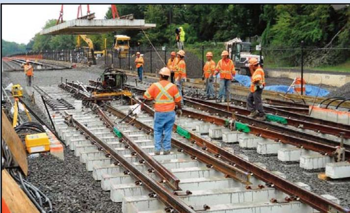
INTO PLACE: Crews lift and place a double crossover panel where existing tracks have been removed. Photo by Stephen Barna, Dulles Corridor Metrorail Project
