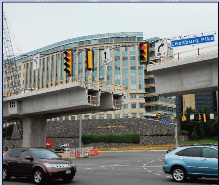
CROSSING GOSNELL/WESTPARK: The cantilevered segmental construction span at the intersection of Route 7 and Gosnell Road continues. Photo by Stephen Barna, Dulles Corridor Metrorail Project
