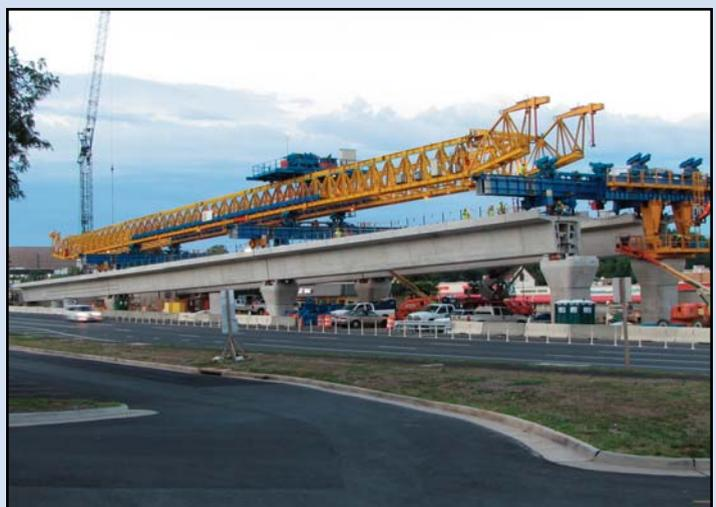
ALONG ROUTE 7: This horizontal crane is building bridges in the median of Route 7 working near the Gosnell/Westpark intersection. Photo by Chuck Samuelson, Dulles Corridor Metrorail Project
