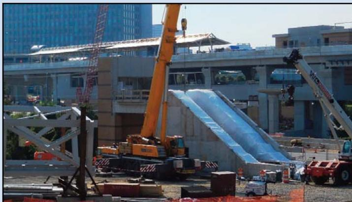
**PEDESTRIAN ACCESS:** Significant progress continues at the pavilion that will contain stairs, escalators and elevators to carry patrons to the Tysons East Station (known officially as the McLean Station). In the background, the framing for the station platform canopy is visible. *Photo by Stephen Barna, Dulles Corridor Metrorail Project*
