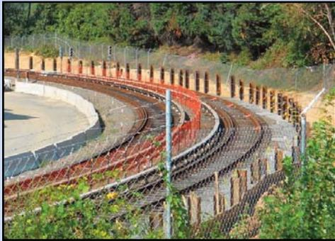
PROVIDING SUPPORT: Piles to support the sound cover box are visible around the edge of the track bed. Photo by Stephen Barna, Dulles Corridor Metrorail Project
