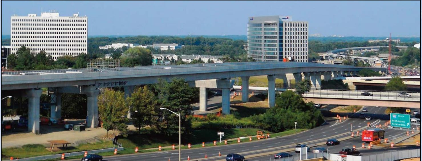
**TYSONS EAST GUIDEWAY FOR RAIL COMPLETED ALONG ROUTE 123:** This view of the Tysons East guideway looking east with Route 123 in the foreground shows the rail bridges (also known as guideway) snaking along the northwest side of the busy highway and crossing Interstate 495. Track installation is complete here. The final precast barrier panels will be installed later this month. *Photo by Stephen Barna, Dulles Corridor Metrorail Project*
