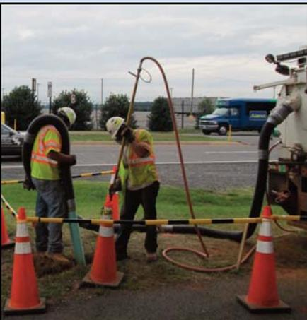
**PHASE 2 UNDERWAY:** Vacuum excavation for utility verification at proposed geotech boring location at the Dulles International Airport. *Photo by Scott Evans, Dulles Corridor Metrorail Project*
