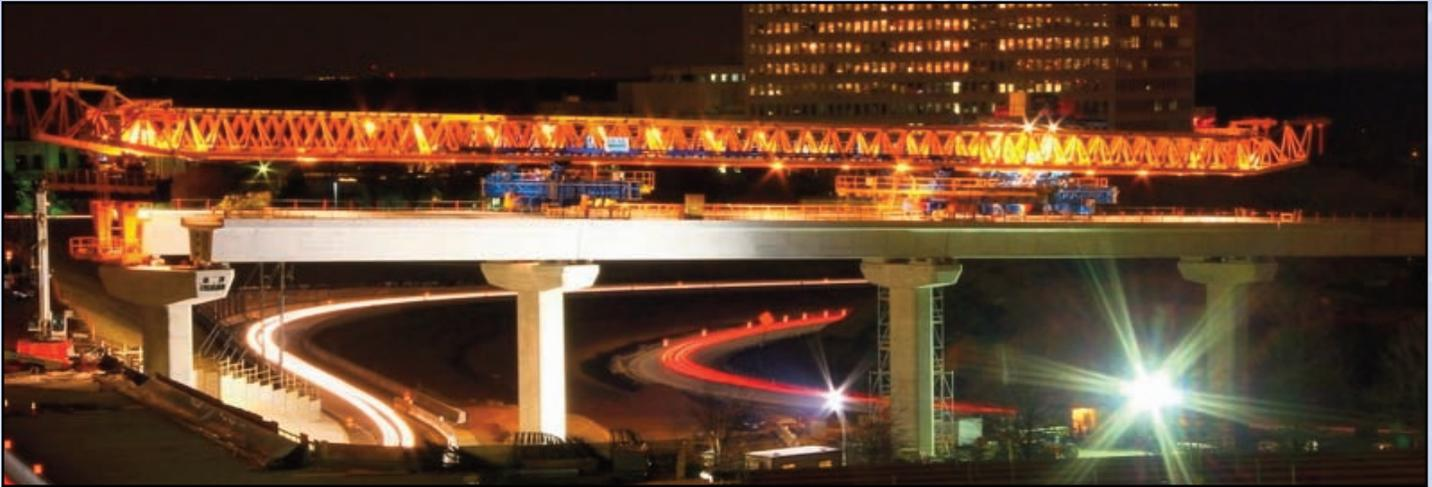
Construction of bridge spans using a giant horizontal crane continues along Route 123 near the Capital Beltway in Tysons Corner
