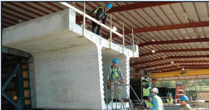
Segments are manufactured off-site at a precast facility near Dulles Airport.
