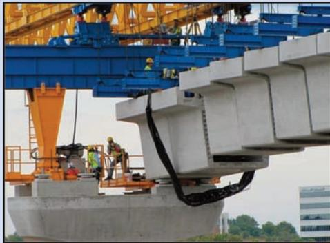
Aerial guideways at I-66 and the Dulles Connector Road where the rail extension connects with Metro's existing Orange Line are being constructed using traditional bridge-building methods.
